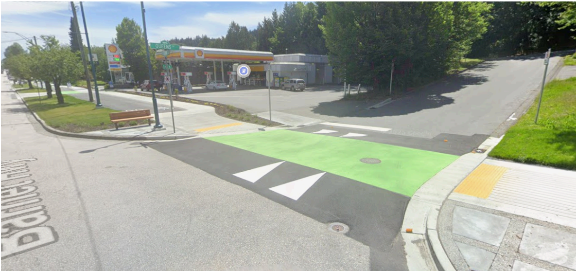
St. John's St. multi-use path in Port Moody, featuring a continuous path with green paint markings
